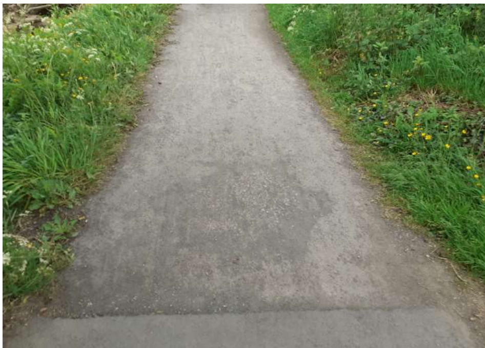
Figure 6-9: Path surface changes from paved to gravel and narrows to approximately 1.5m width
